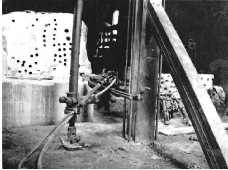
IR #248 Drill in position.
