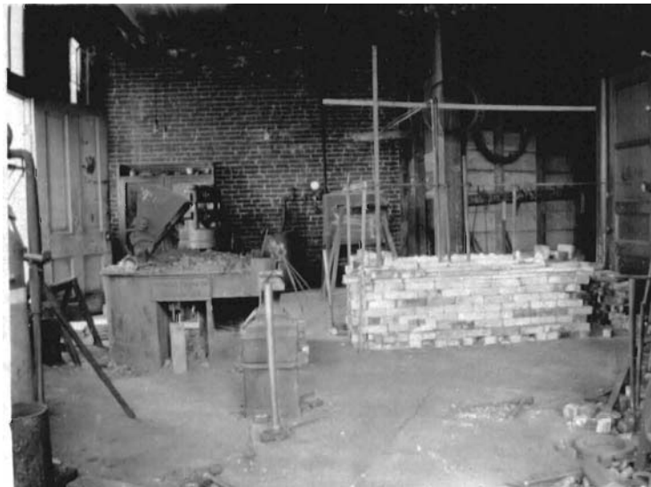
General view of sharpening shop.
